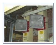
**Note:** If explosion relief vents through a roof then consideration should be given to the potential for snow or ice accumulation in colder periods and water building-up in heavy rain. This will have an impact on the effectiveness of the relief device.
